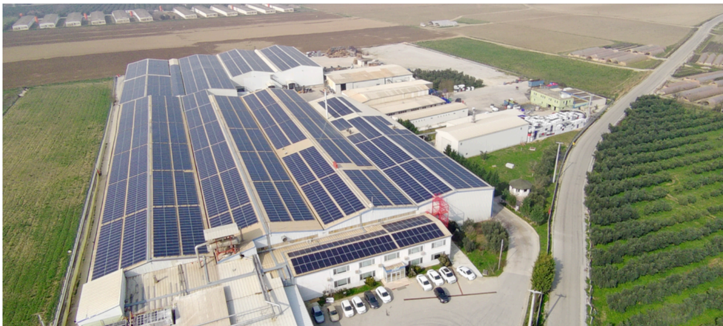
NAMSAL PRODUCTION FACILITY · ORHANGAZI, BURSA
